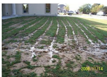
Examples of failing leachfields. The majority of failing systems are identified by surface effluent (middle and far right). However, the majority of failing systems are not evident to the naked eye and may appear as a green lawn (left)
