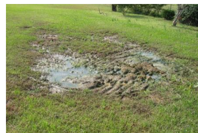
Examples of failing leachfields. The majority of failing systems are identified by surface effluent (middle and far right). However, the majority of failing systems are not evident to the naked eye and may appear as a green lawn (left)
