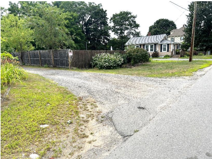
Dickey Street. Looking west towards the northern site entrance and Tax Map 10 Lot 110. (8/6/2025)
