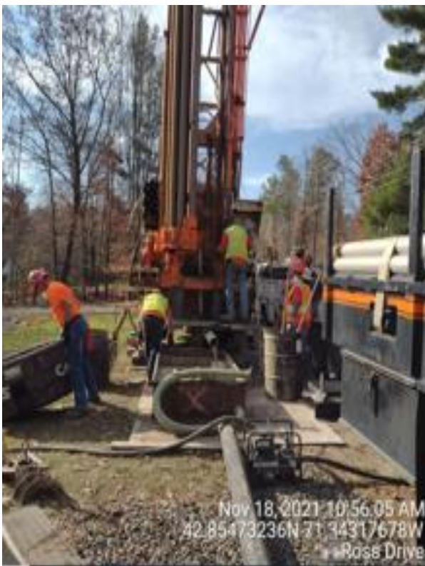
Figure 1: Contractors setting up a drill rig.
