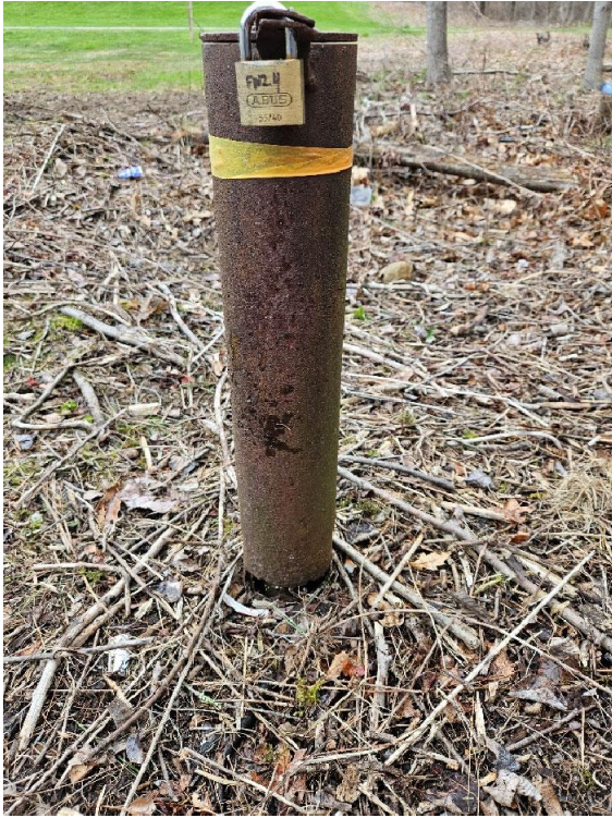
Photo 5: Damaged/corroded casing at base of FW-24
