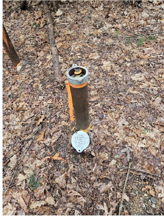
Photo 2: Unsecured well with unsealed well cap
