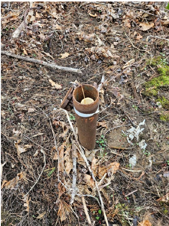
Photo 3: Unsecured well with unsealed well cap
