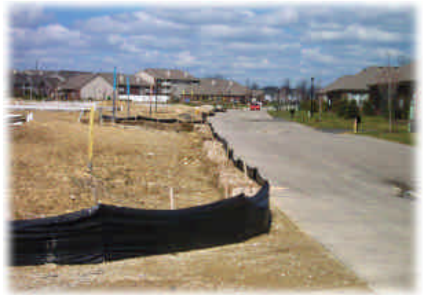
Low impact development – stormwater runoff from construction activities can have a significant impact on water quality so protecting a site during construction is critical
