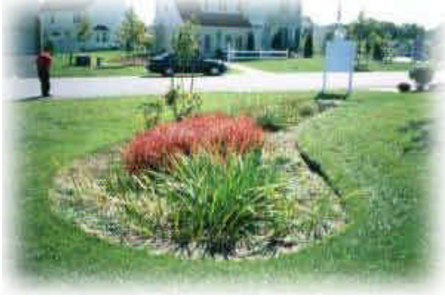
A bio-retention cell: Planted in low-lying areas, the gardens contain specific layers of soil, sand, and organic mulch. These layers naturally filter the site's runoff, substantially reducing common homeowner pollutants such as lawn fertilizers and driveway oils and providing protection for the receiving waterways. Source: Low Impact Development Center, Inc.
