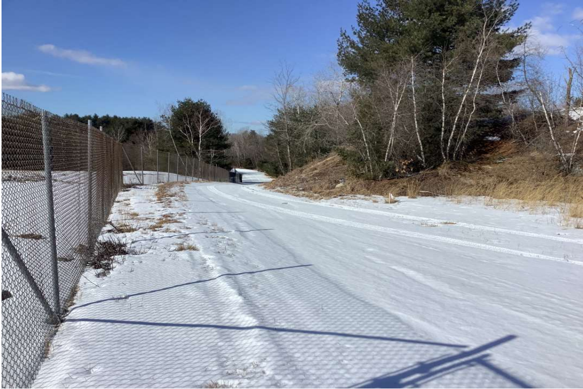
Photo No. 51: SWLF – Access Road (View: Northwest)
