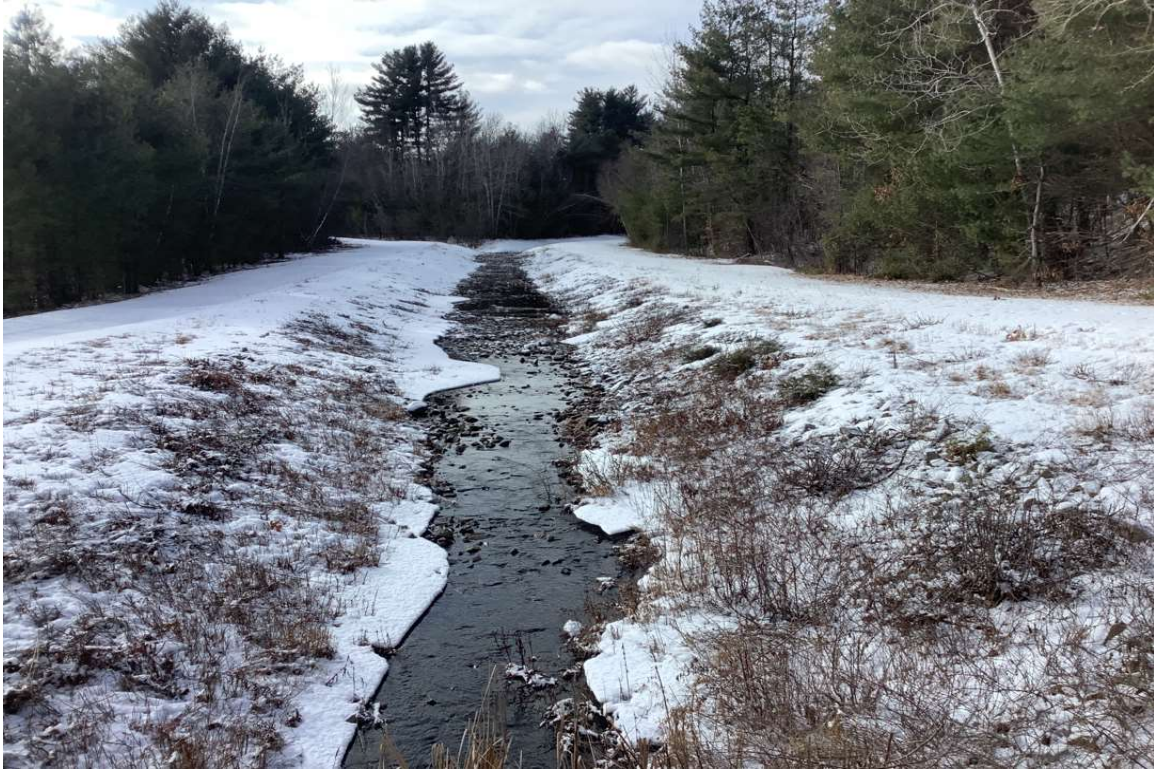
Photo No. 4: Swale F (View: South)
