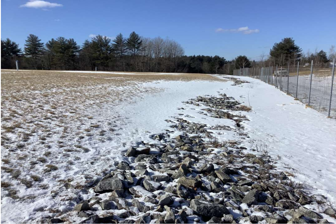
Photo No. 65: SWLF – Northern Toe-of-Slope (View: Northwest)
