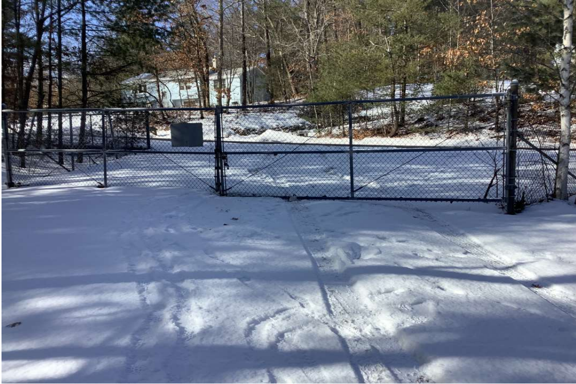
Photo No. 12: Access Road Entrance Gate (View: West)
