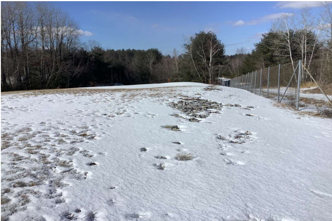
Photo No. 52: SWLF – Northern Toe-of-Slope (View: Northwest)
