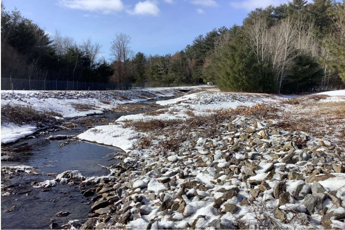
Photo No. 8: Swale B, sediment and vegetative build-up removed by Town (View: Southwest)
