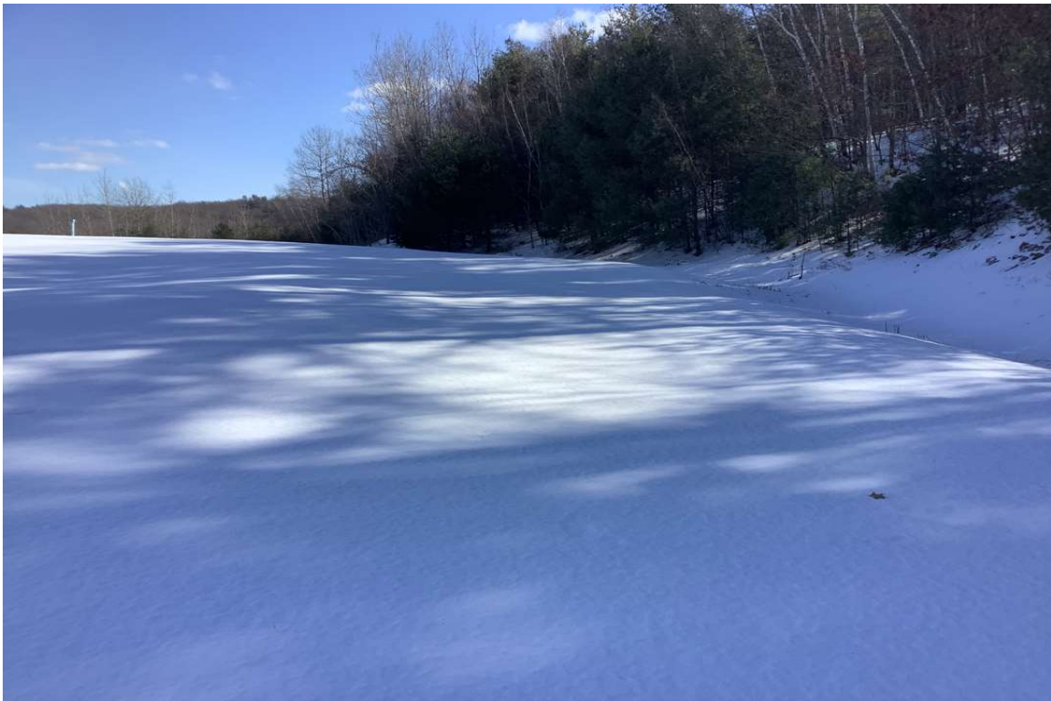
Photo No. 56: SWLF – Southern Toe-of-Slope & Surface (View: East)
