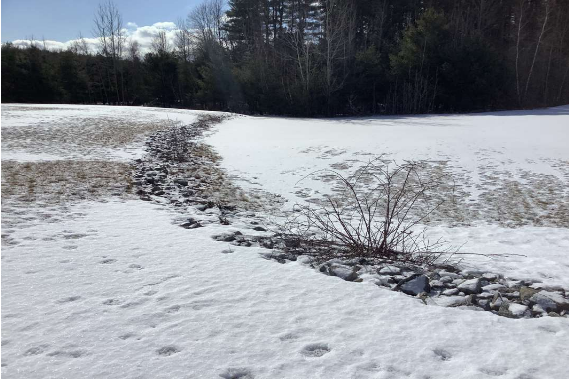
Photo No. 30: Town Dump – Southern Toe-of-Slope (View: Southeast)
