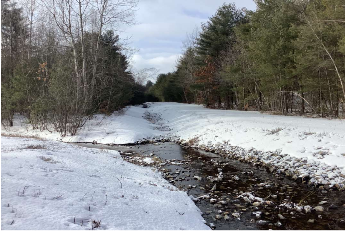
Photo No. 1a: Confluence of Swale E & H (View: Southwest)
