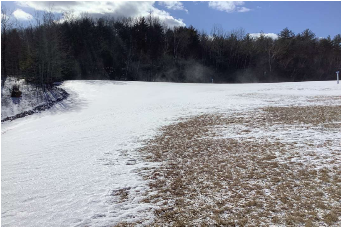
Photo No. 62: SWLF – Eastern Toe-of-Slope (View: North)
