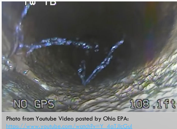
Water entering a well from fractures (cracks) in the rock
